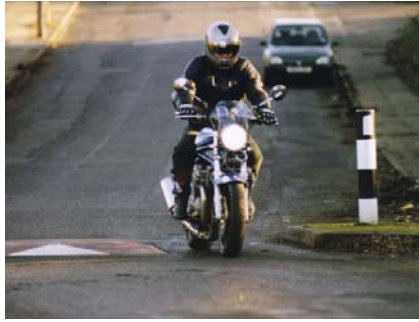
Build outs in association with traffic calming should be conspicuous. Keith Sharples Photography.
