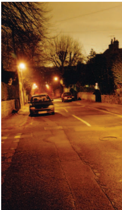
Broken and patched surface near to traffic calming. Keith Sharples Photography.
