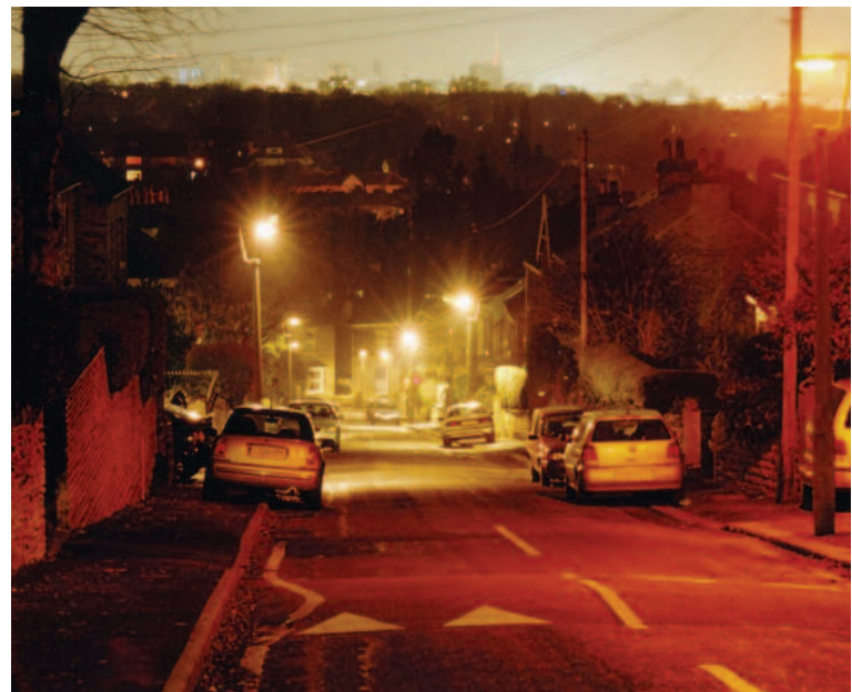
Poorly lit traffic calming presents a hazard to all users, but in particular motorcycles. Keith Sharples Photography.
